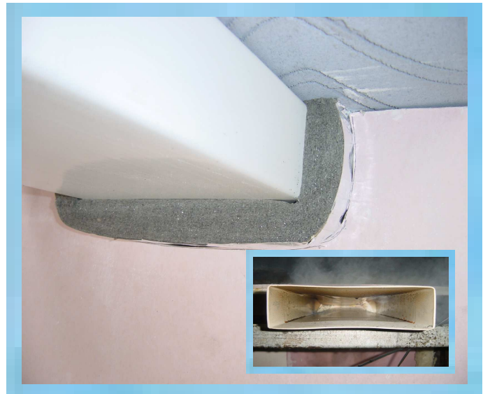
Vent Duct Fire Sleeve Installed Under Ceiling Soffit Inset shows Duct sealed by the Fire Sleeve in a Fire
